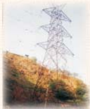
220 kV D/C TL Tower, Abu Dhabi
