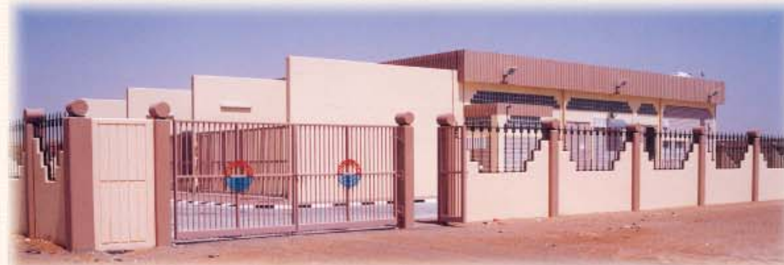
33/11 kV GIS Substation at Al-Ain, UAE
