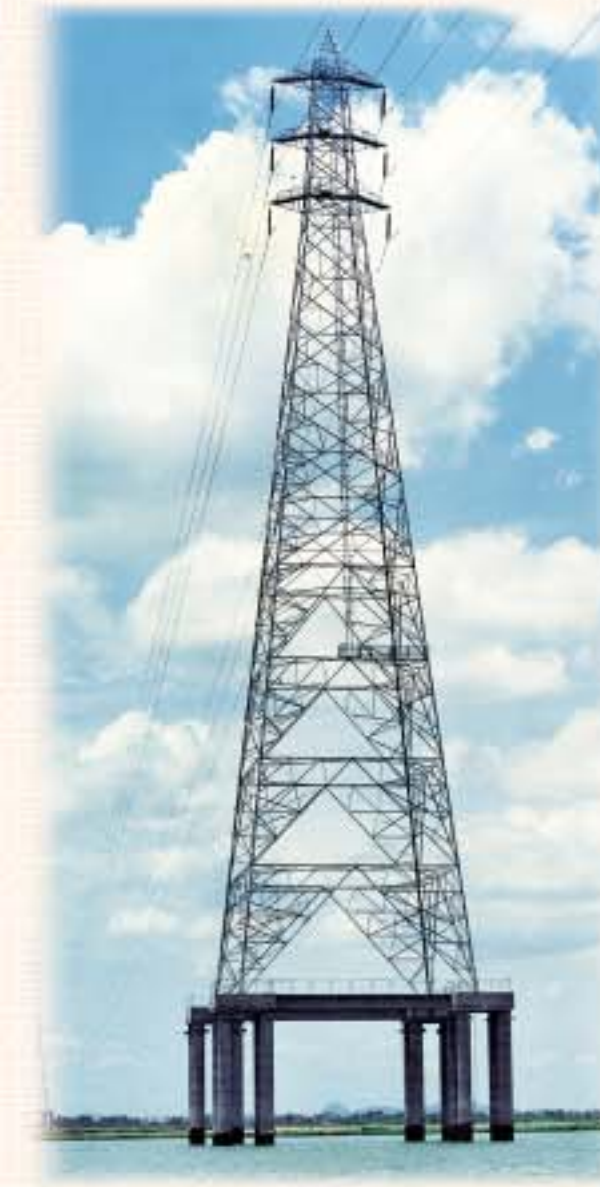
220 kV 'Krishna' river crossing TL tower, India
