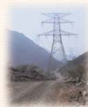
400 kV D/C TL at Fujairah, UAE
